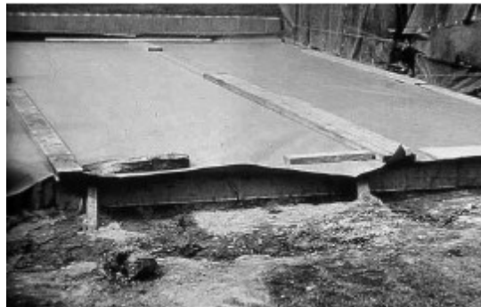
Slab-on-grade covered with waterproof paper
