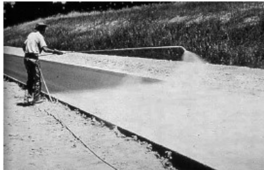
Application of liquid-forming compound with hand sprayer.
