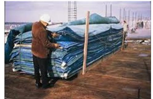
The ready-mix concrete producer and control concrete temperature and furnish concrete to comply. Concrete temperature should not exceed these values by more than 10°C. Concrete at a higher temperature requires more mixing water, has a higher rate of slump loss, and is more susceptible to cracking. Concreting in cold weather provides the opportunity for better quality, as cooler initial concrete temperature will typically result in higher ultimate strength and improved durability.
