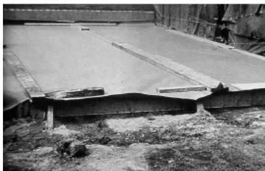
Slab-on-grade covered with waterproof paper
