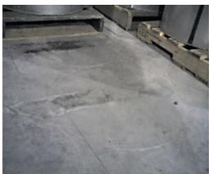
Factors found to influence discolouration include: calcium chloride admixtures, variations in cement alkali contents, delayed and uneven hydration of the cement paste, admixtures, hard-troweling of concrete surfaces, inadequate or inappropriate curing, concreting practices and finishing procedures that cause variations in the water-to-cementing materials ratio at the concrete surface, and changes in the concrete mix design proportions or constituents.
