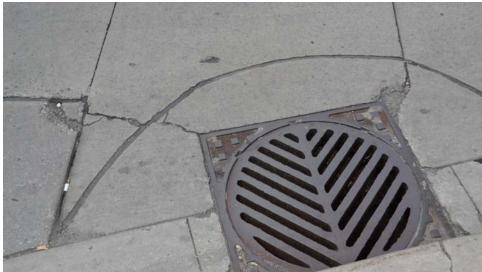
FIGURE 8 Cracking near catchbasin.
