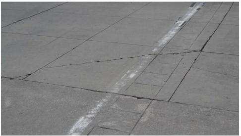
FIGURE 9 Cracked slabs in crosswalk area.
