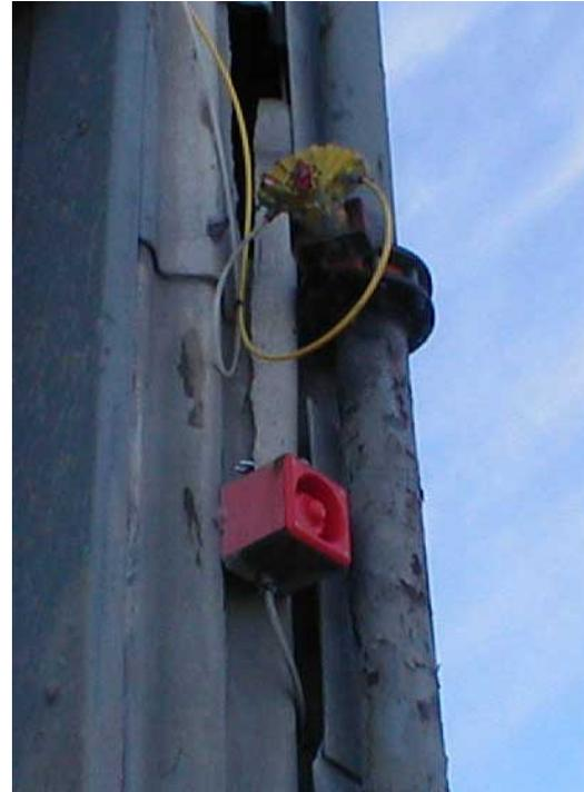
**Figure 5.** Shut-off valve, located mid-pipe, and alarm to indicate activation of system.
