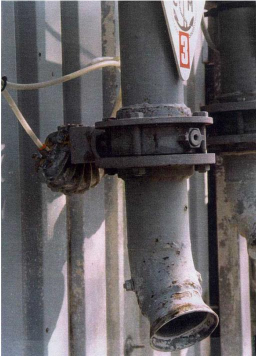
**Figure 4.** Shut-off valve located close to connection point, which is labelled.
