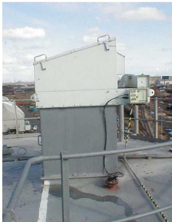
**Figure 2.** Filter housing on top of silo installation.
